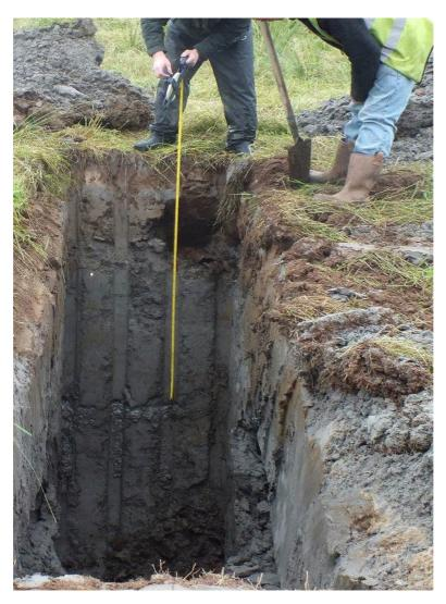
A number of test pits were dug (see picture above) to study soil profiles and get an understanding of drainage problem.
