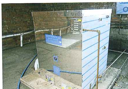
The hot water tank may be well insulated, but no lagging on the pipes will detract from the overall efficiency of the system.
