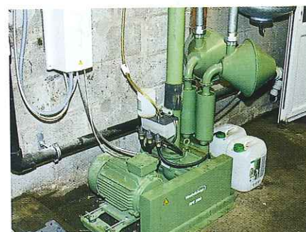
A vacuum pump that alters its speed in respect of demand consumes less electricity than those that work at a constant speed.
