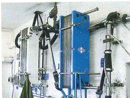
Milk cooling costs can be pegged through the use of plate heat exchangers. The payback period, in some cases, can be less than a year.
