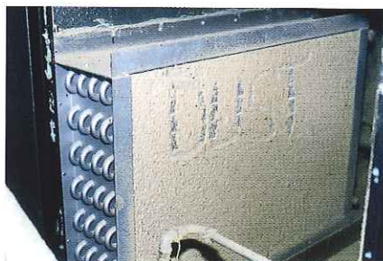
Dust on the intake of refrigerator systems drastically reduces the efficiency of the unit and means it has to run for longer periods.
