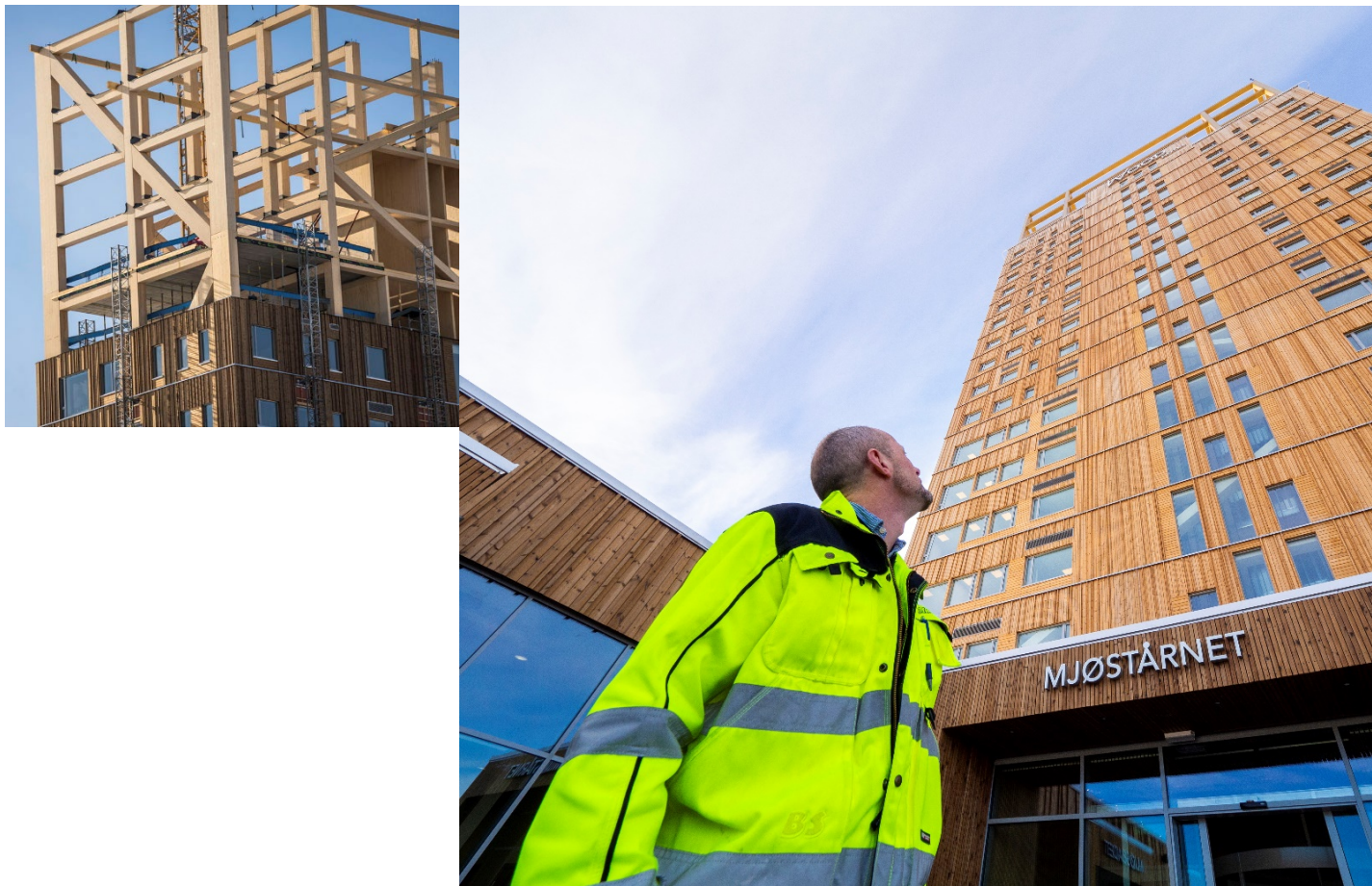
Plate 6: Mjøstarnet, in Brumunddal, Norway, the tallest wooden building in the world and (inset) Glulam engineered construction components. (Source: Moelven.com )
