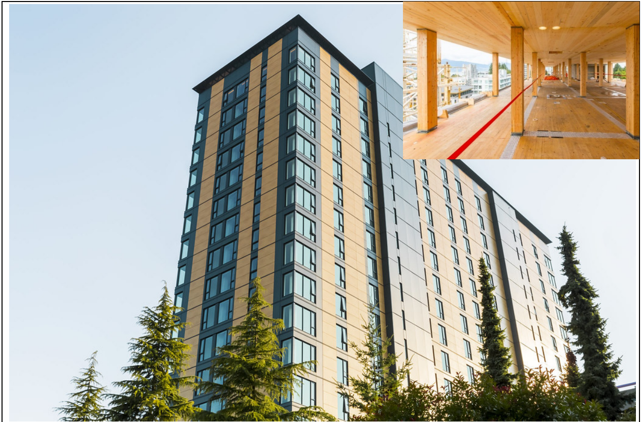
Plate 7: Brock Commons Student Residences in the University of British Columbia, Vancouver which (inset) uses CLT floor panels and Glulam Columns (Source: Harte. NUIG)
