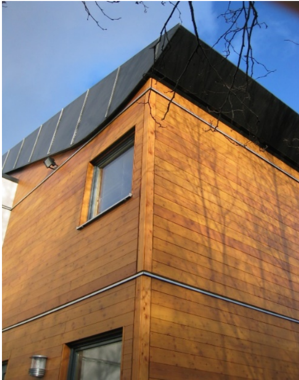
Plate 2: Decorative cladding (Source: Source: FII )
