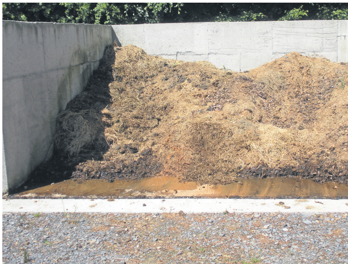
Manure pit with channel to divert effluent to underground tank Wendy Conlon
