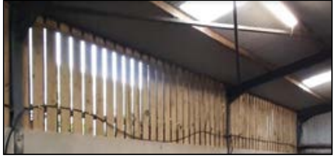
Figure 1. An example of Yorkshire boarding being used as an inlet in calf housing
