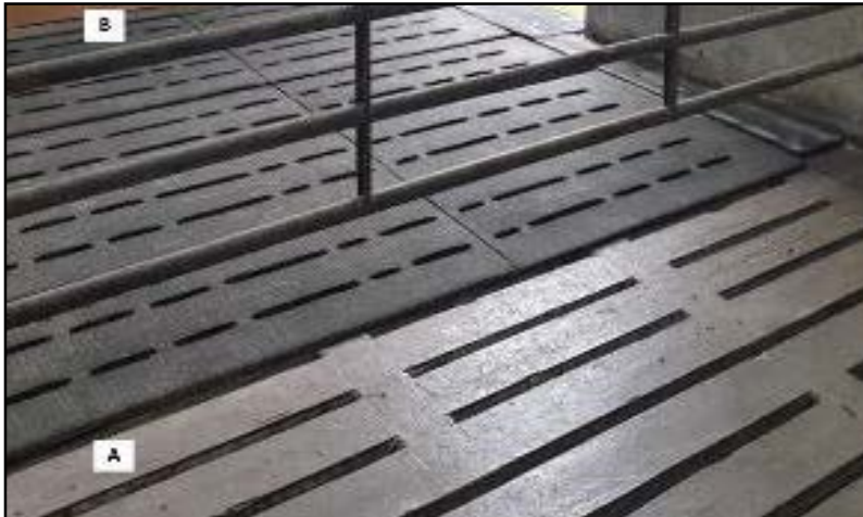
Figure 1. Photograph showing (A) concrete slatted floor pen (CS), and (B) the concrete slats overlaid with rubber mats (RM)
