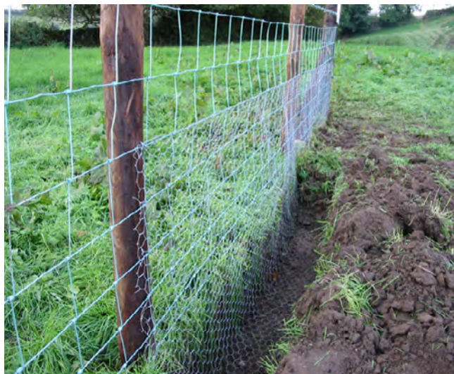
This sturdy fence will protect trees from livestock. Note the rabbit wire buried and bent outwards.
