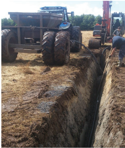
Figure 26. Drainage work at Crossmolina, Co. Mayo
