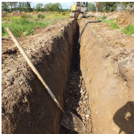
Figure 11. Drainage trench excavation
