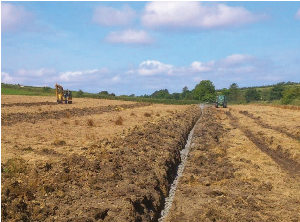
Figure 22. Drainage Work at Kishkeam, Co. Cork
