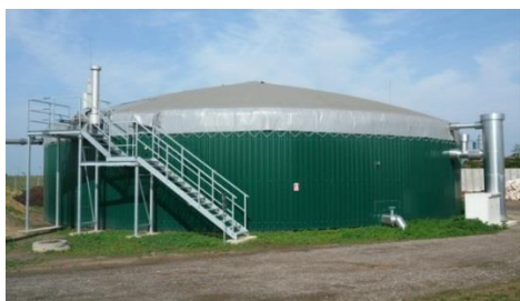
Anaerobic digester converting spent mushroom substrate into biogas, heat and fertilizer (Source: www.pleurotus.hu )
