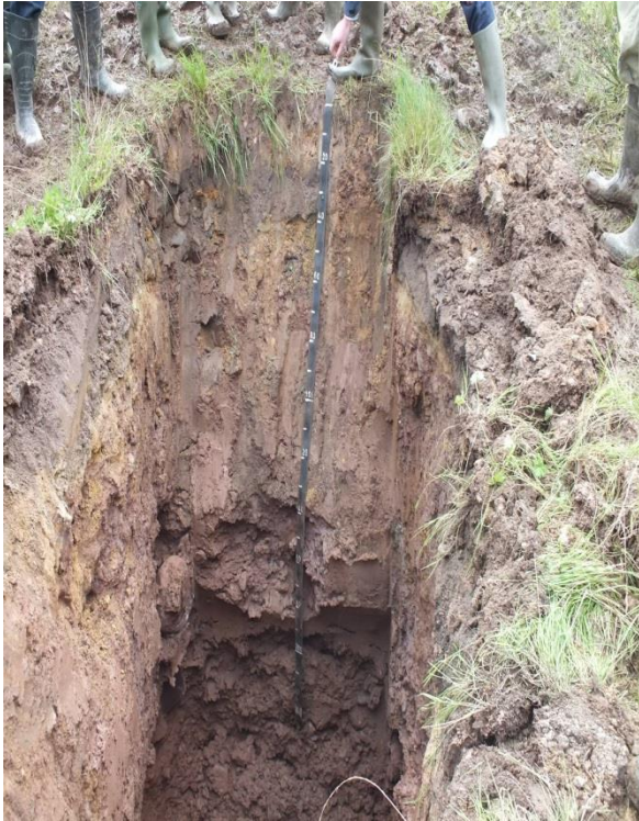
Soil Test pits
