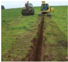
Fig 1b. Drainage trench excavation
