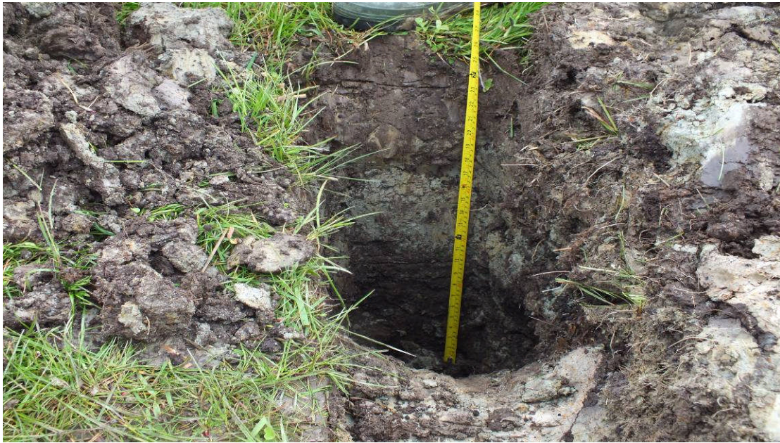
Picture 2 Naked mole installed at 450 mm
