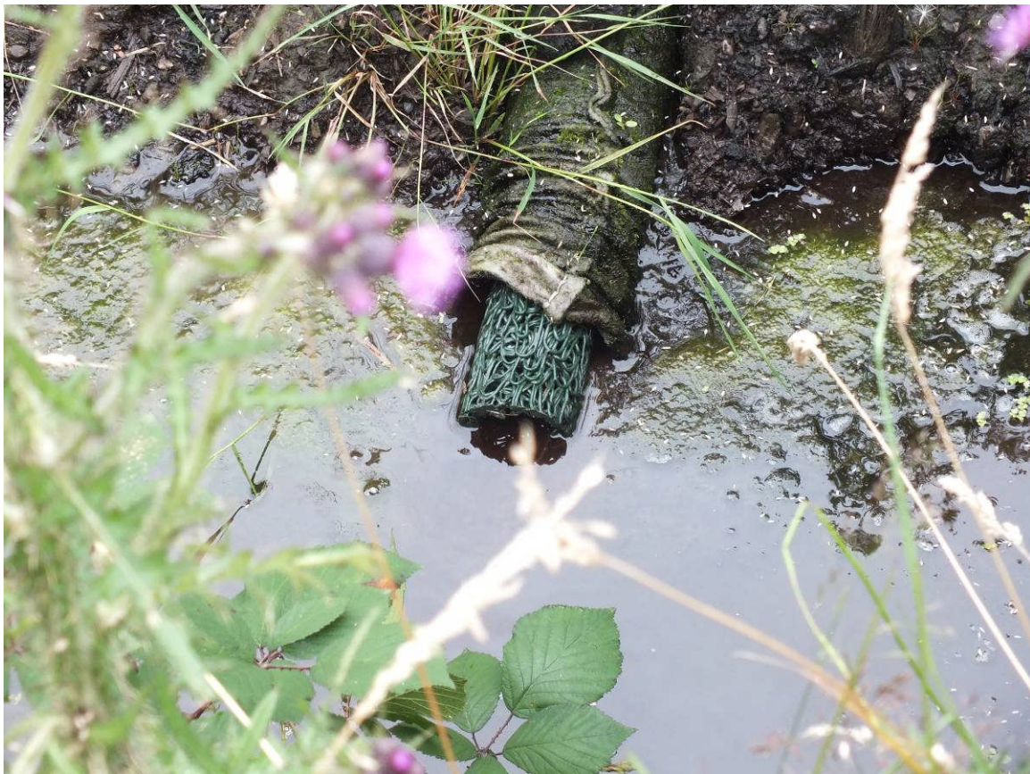
Picture 2: Connacht Agri pipe with filter around it
