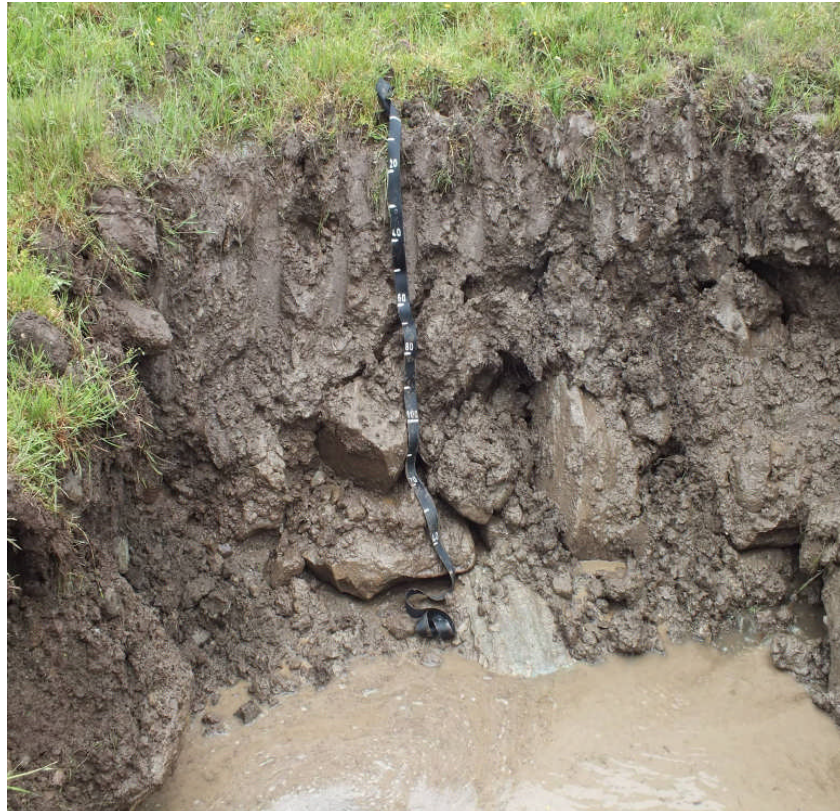
Picture 3 which was taken in Paddock 19 is an example of the type of drains that were installed on the farm. The large stones that can be seen around the tape were used to fill the drain. There was a very good flow of water in this drain.
