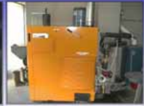
KWB 20kW Log Boiler, Strabane
