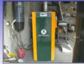
KWB 20kW Log Boiler, Strabane
