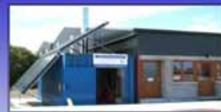
150kW Multi Fuel Biomass, 20kW Solar, Co. Louth
