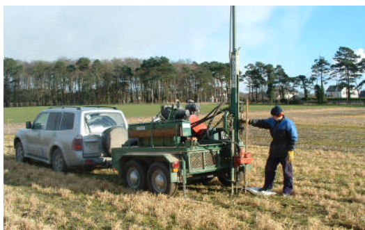
Installing groundwater investigation wells.
