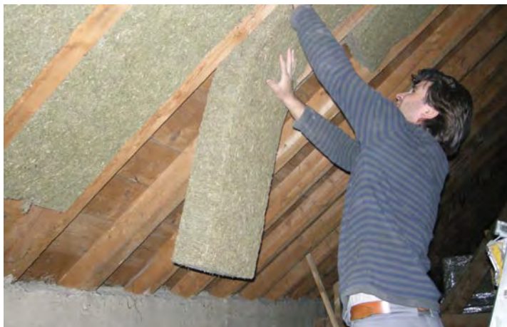
FIGURE 1: Installation of insulation boards made from grass fibre (Source: Stefan Grass; www.gramitech.ch ).
