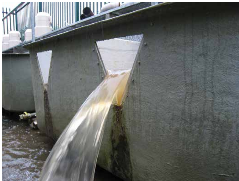
Figure 1. Tanks, V-notch weirs and automatic samplers installed at the bottom of grassland plots to monitor water volumes and nutrient losses in overland and subsurface drainage flow.
