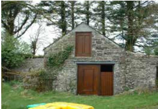
Figure 2: Repaired farm building
