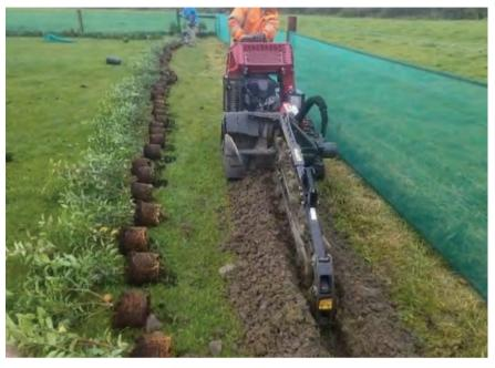
A trencher poistioned 1.2m away from boundry fencing planting 3 Lt potted prunus with a windbreaker attached to the boundary fence.
