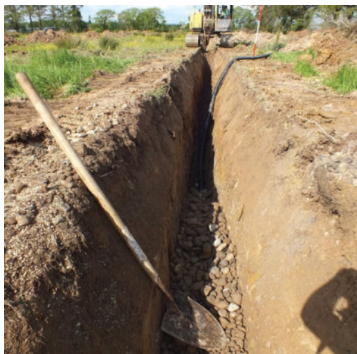
Figure 11. Drainage trench excavation
