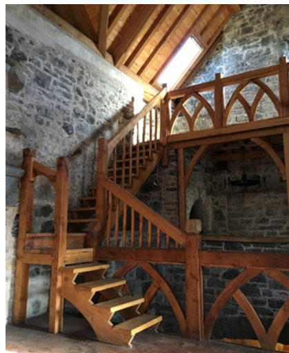
Interior of Springfield medieval tower refurbished using local oak. \Mark Moore
