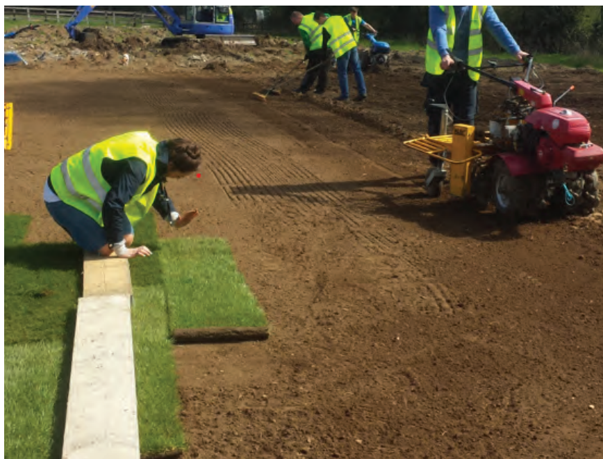
The turfing process: work forwards from planks on top of the turves just laid.
