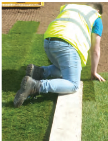
The turfing process: work forwards from planks on top of the turves just laid.
