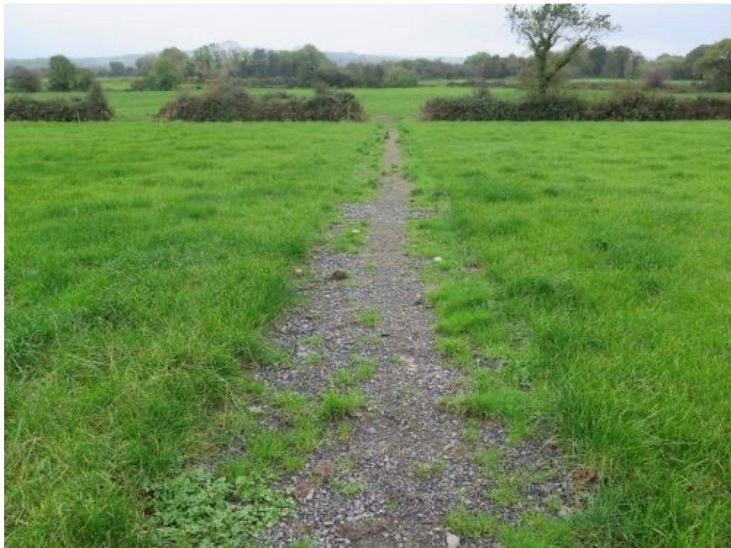
Image 1. Permanent un-fenced spur roadways installed
