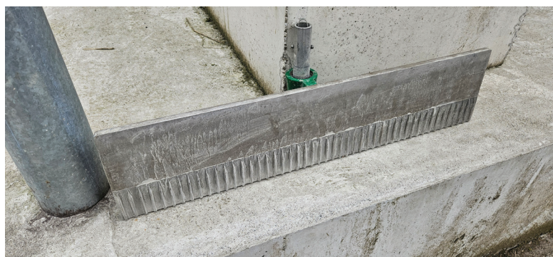
Figure 6 shows a suitable concrete finish (for passageways) produced by the 'bullfloat' on the right Figure 7 The grooves are parallel with the long axis of the building and the scraper track. The concrete surface is level, the grooves are close and have well defined edges. It is often recommended to have the grooves at right angles to the main direction of animal movement, this is not the case here but the density and quality of the grooving will compensate. This grooving will provide good support to cows backing out of cubicles.
