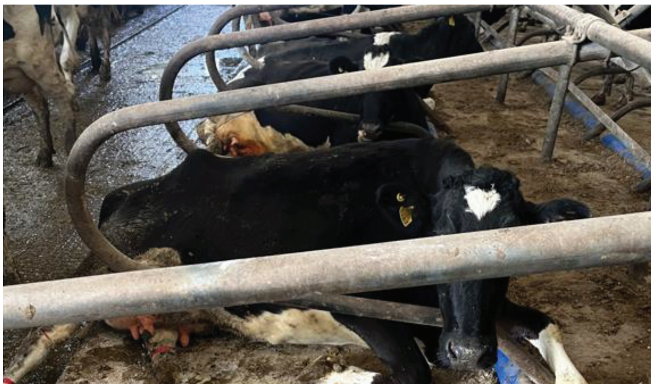
Figure 3: Cows stretched out & comfortable (the kerb is 150mm high excluding the mat and the brisket pipe is 100mm in diameter, both facilitating cows that want to stretch out).
