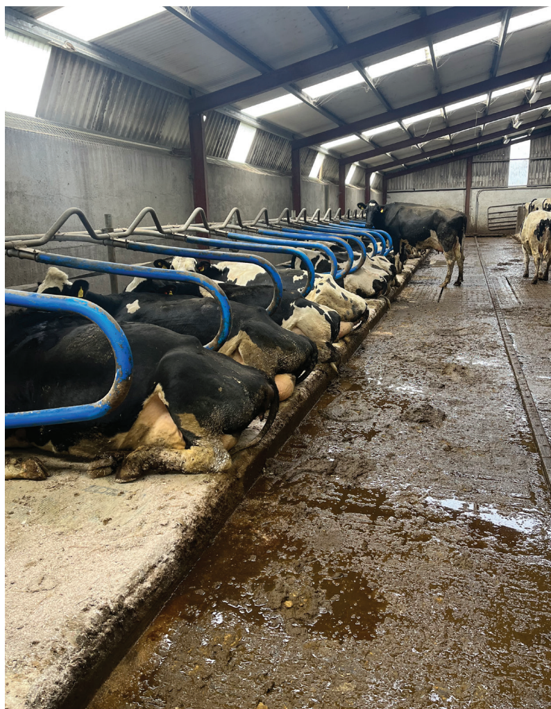
Figures 10 & 11: Looped neckrails and partially plastic cubicle divisions
