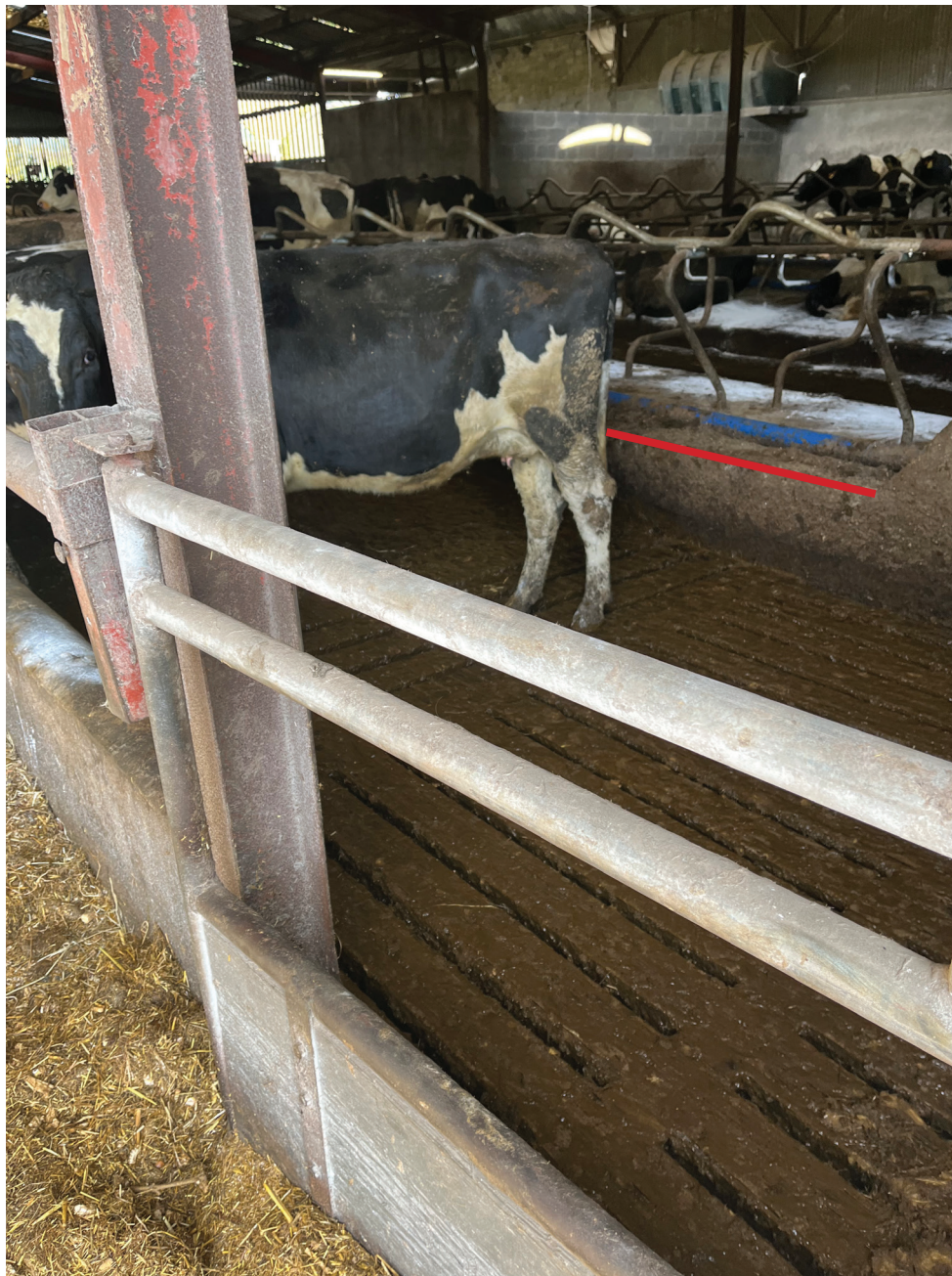
Figure 17: Old cubicle houses can be improved, a wall in front of the cubicles has been removed (where red line is) and a looped neckrail installed. In this situation a band or an extra bar maybe needed to stop animals attempting to walk through the cubicle.
