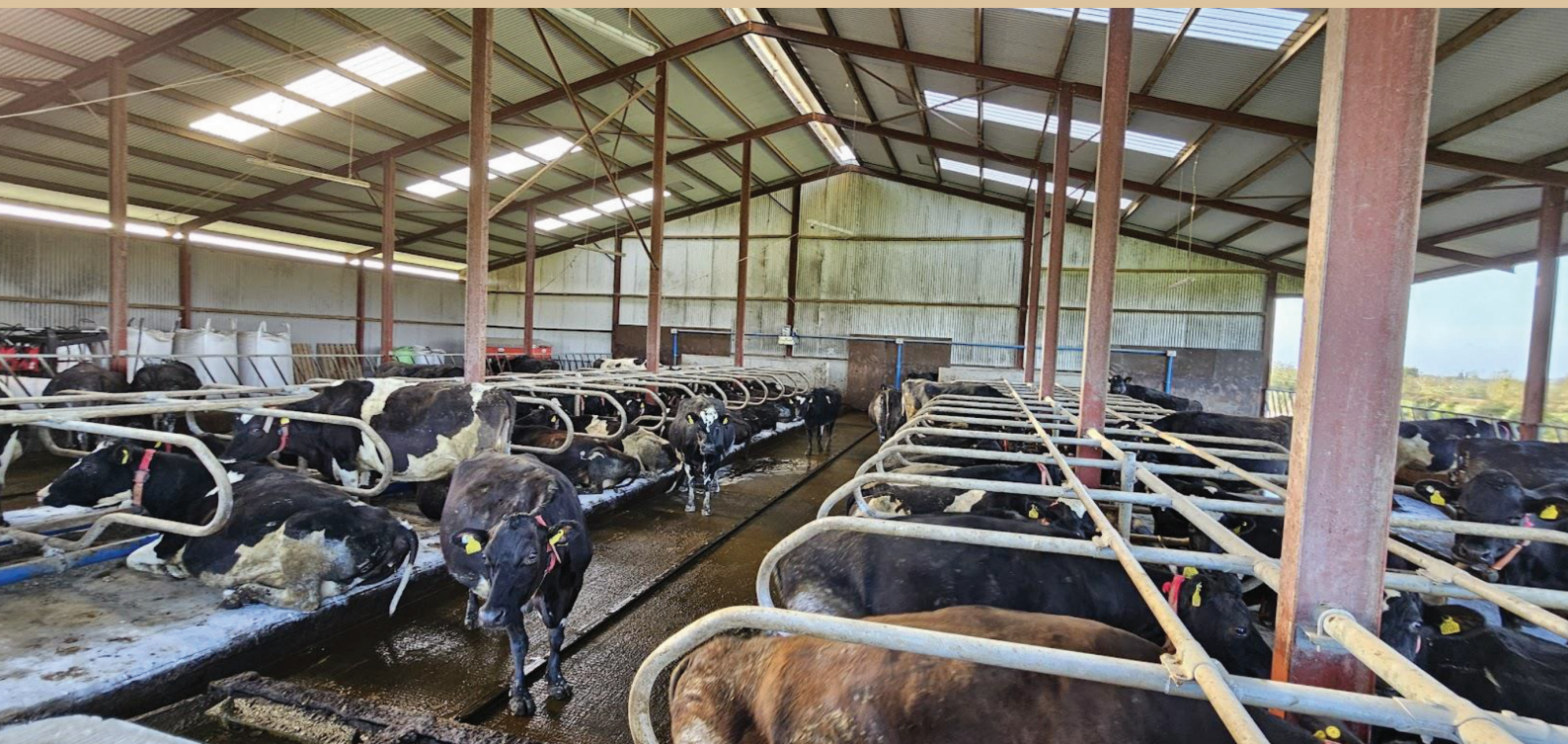
Figure 5: 500kg cows on average in head to head cubicles that are 4.3m (two x 2.15m cubicles) long. These cubicles are very comfortable with a high level of occupancy. They are however, too short for bigger cows. High yielding cows (kgs fat & protein) will be 'big' in terms of body capacity so the width of the cubicle is also important.
