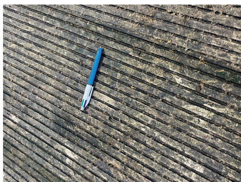
Figure 6 shows a suitable concrete finish (for passageways) produced by the 'bullfloat' on the right Figure 7 The grooves are parallel with the long axis of the building and the scraper track. The concrete surface is level, the grooves are close and have well defined edges. It is often recommended to have the grooves at right angles to the main direction of animal movement, this is not the case here but the density and quality of the grooving will compensate. This grooving will provide good support to cows backing out of cubicles.
