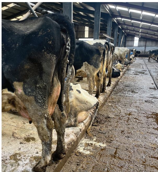
Figure 3: Cows stretched out & comfortable (the kerb is 150mm high excluding the mat and the brisket pipe is 100mm in diameter, both facilitating cows that want to stretch out).
