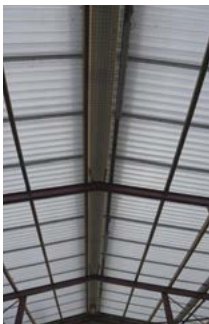
Roof sheeted with clear polycarbonate sheeting to improve brightness in the shed.
