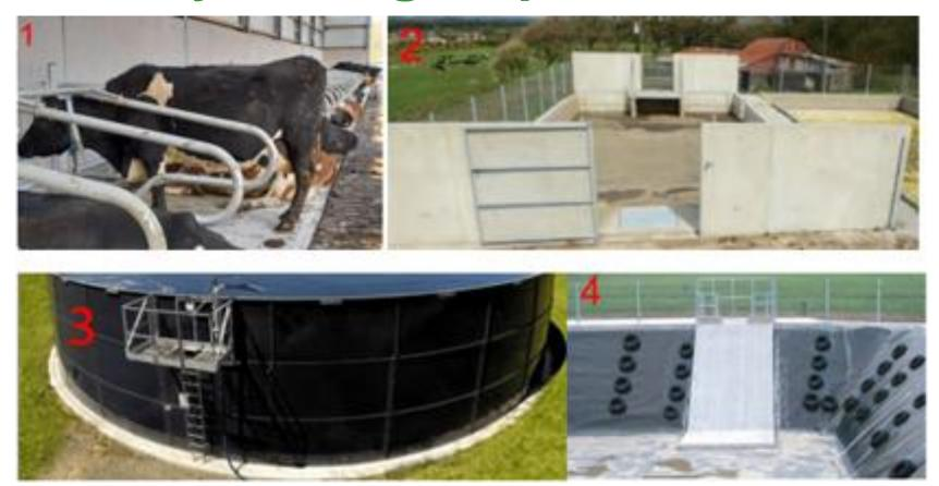
The above pictures show 4 common storage options: 1 is a slatted tanks, 2 is an underground concrete tank, 3 is an overground steel tank and 4 is a lined lagoon
