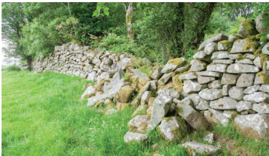
Wall in need of repair. Photo courtesy of the DSWAI.
