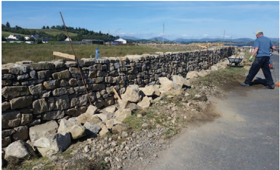
Section of Famine Wall at Salt Hill Pier in Co. Donegal. The wall and pier were built as poverty relief work in 1846, but the wall fell into disrepair. Photo by Louise Price via Tír Chonaill Stone Festival.
