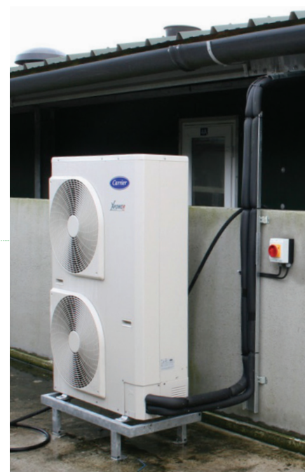
Heat pumps capture energy in the air, ground or water and deliver it to buildings.
